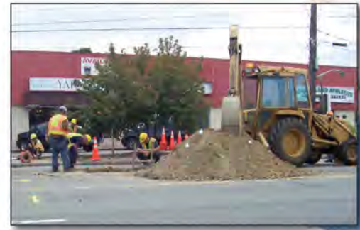
SFWD crew hard at work repairing a water main.
