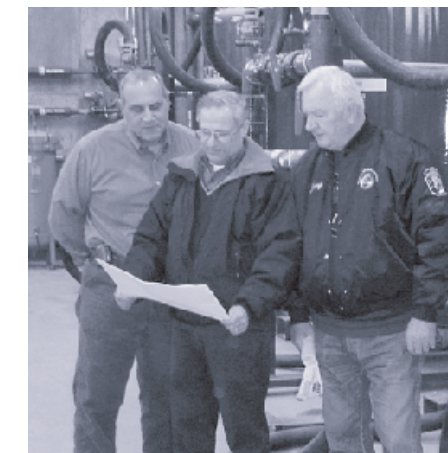
SFWD commissioners tour Liberty filtration facility.
