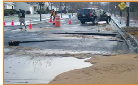
SFWD team arrives on scene within 30 minutes to repair water main break
