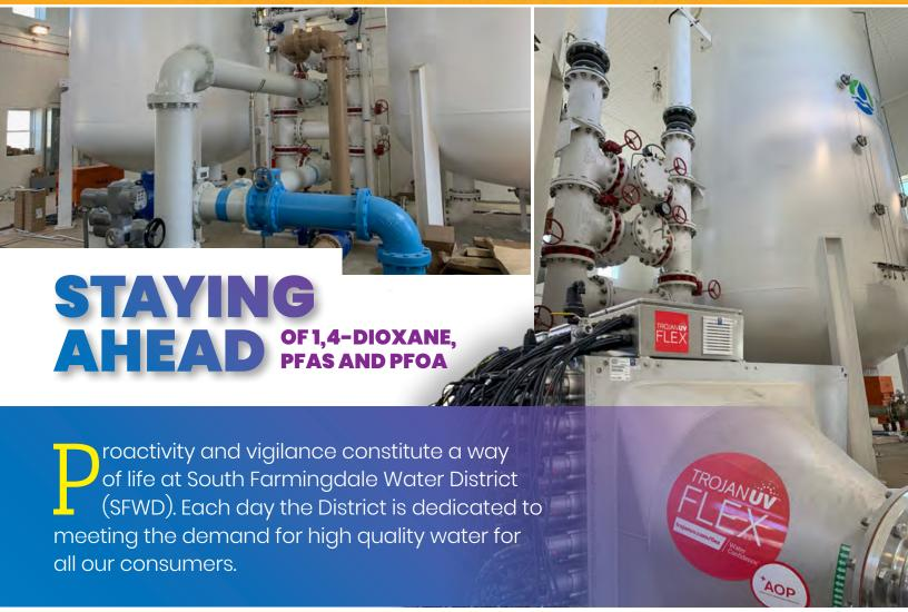
Advanced Oxidation Process (AOP), which is the most technologically advanced and proven solution to remove 1,4-dioxane from drinking water, was pilot tested at Plant No. 3 back in 2019. Our new AOP system has now recently been installed and will be fully operational this summer. Plant No. 3 had been offline since 2018 and will be in full compliance with all local, state and federal regulations.
