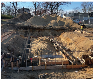
Construction of Plant 6 has begun. Footings for foundation in place.
